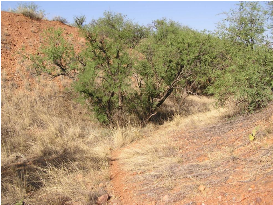
Figure 4. CCC-constructed earthen dam, CCC Canyon, Patagonia. (S.E. Hunt)
